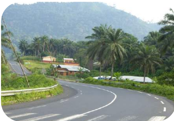
1 - Supporting infrastructure development
